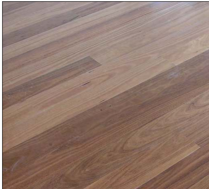
Engineered floor laid on acoustic underlay
