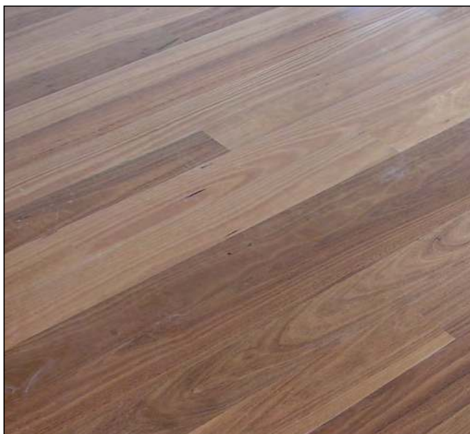
Engineered floor laid on acoustic underlay
